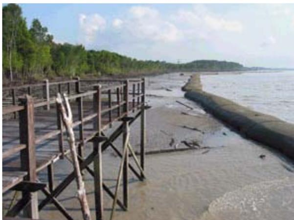
*Installation of geo-tube as wave breaker in Tanjung Piai by Drainage and Irrigation Department*
