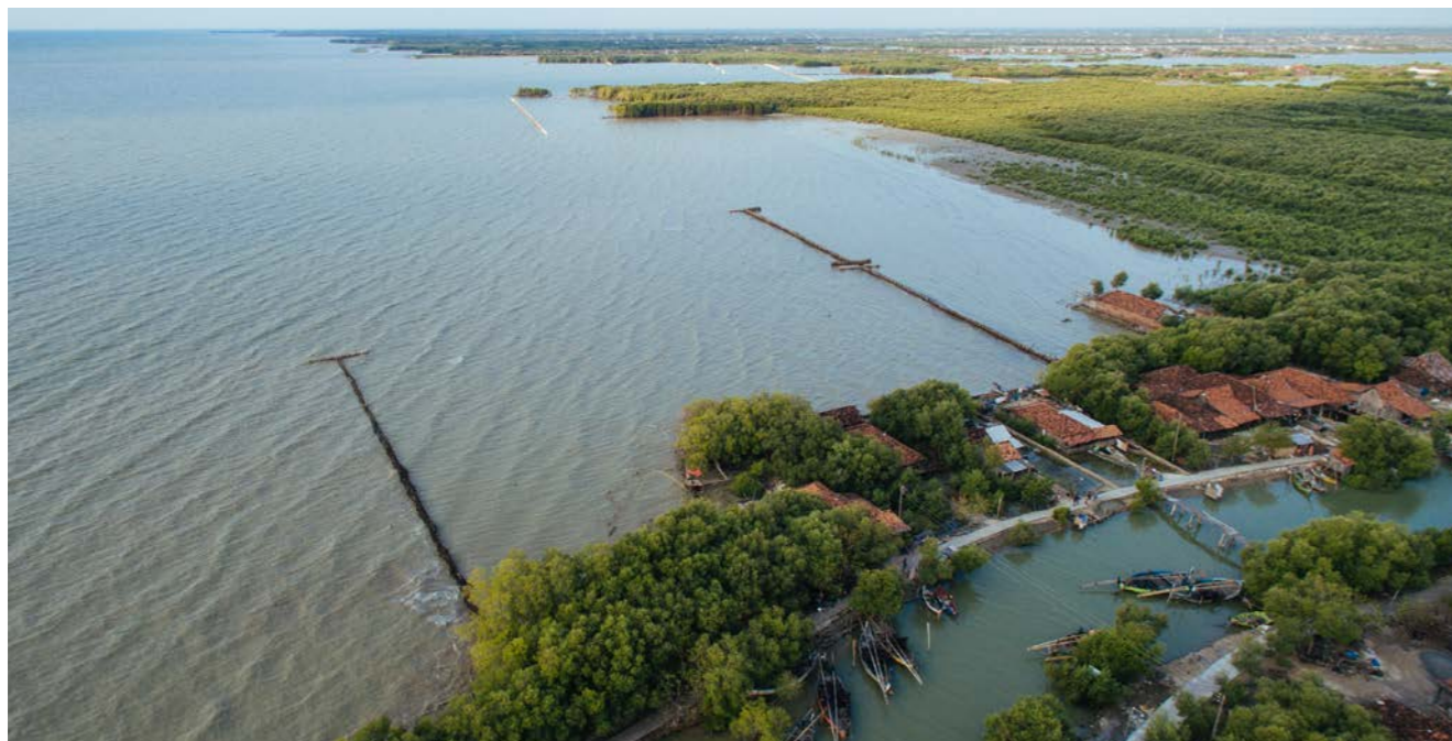
Permeable Structures in Bedono Northern Java, Indonesia.
