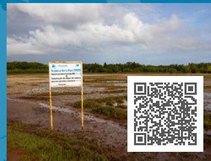
Guinea-Bissau Restoration work
