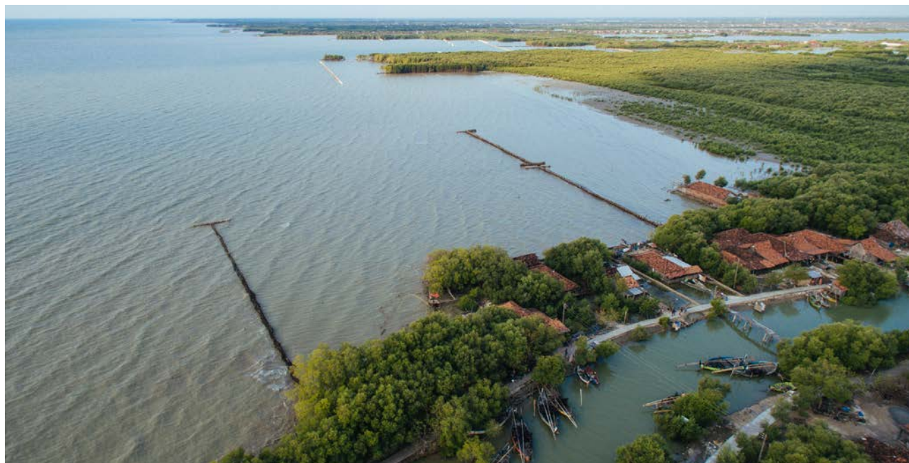
Permeable Structures in Bedono Northern Java, Indonesia.
