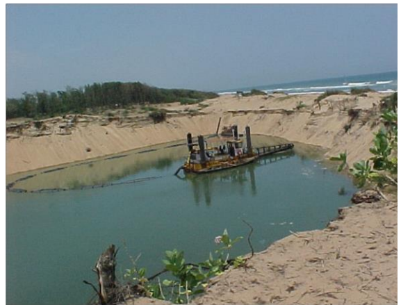
Figure 18: Chilika artificial mouth opening by engineers
