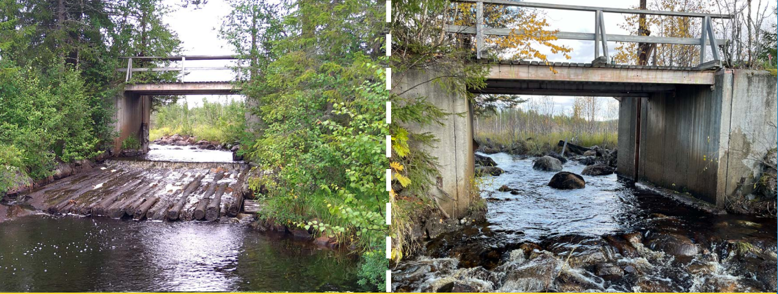
FRÄKÄNTJÄRNSDAMMEN TIMBER FLOATING DAM – VINDEL RIVER CATCHMENT – SWEDEN © Rewilding Sweden ( link )
