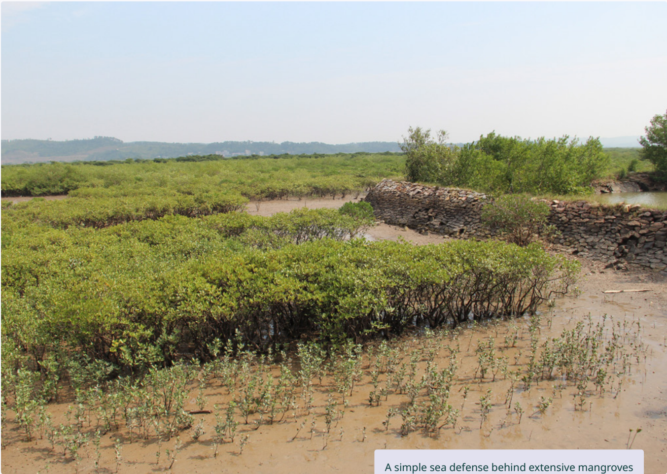
A simple sea defense behind extensive mangroves in southern China. © Mark Spalding / TNC
