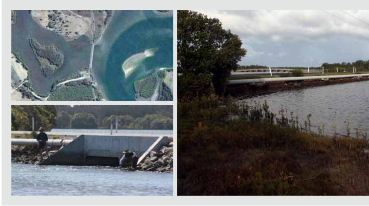
improve ecological processes in the lower Clarence estuary. In 2006, after years of consultation, geotechnical studies and extensive stakeholder engagement, WetlandCare Australia initiated the installation of a large doublecell box culvert. This design allowed the greatest volume of tidal exchange and the best access for fish passage.
