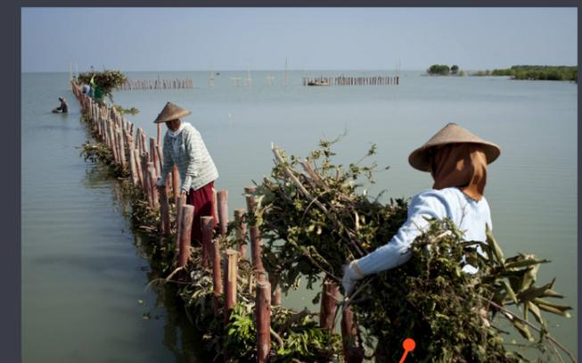
In Java, Indonesia, permeable dams are being used to retain sediments and allow natural mangrove recovery
