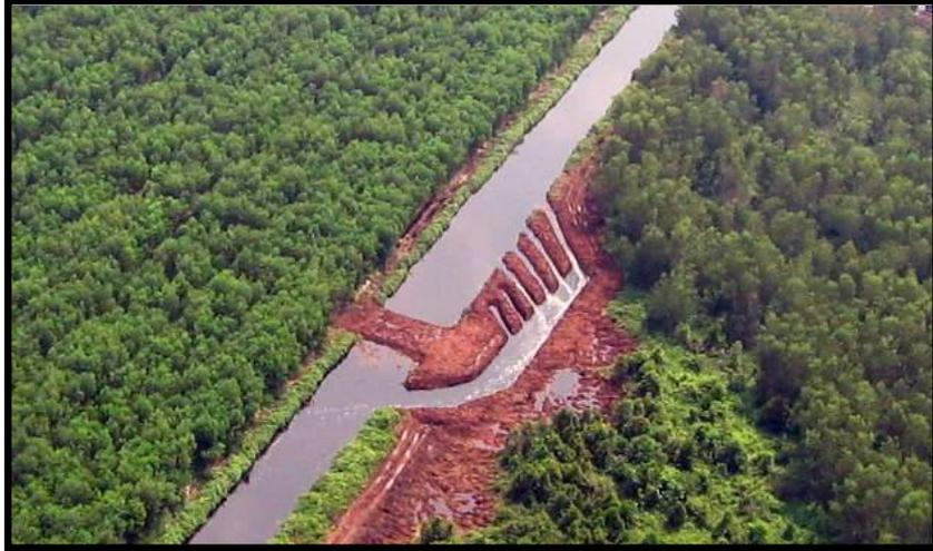
*Figure 6 Example of APRIL Operations dam and bypass structures (2 still under construction) in a plantation canal. The main canal is closed with a peat dam, and water diverted around it through bypasses in which water levels can be controlled. A spillway (not shown) has now been added to this design, and dimensions have been modified to achieve greater robustness under extreme flow conditions.*
