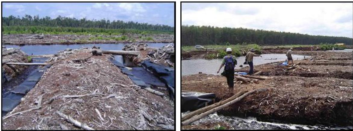
*Figure 7 Example of APRIL Operations bypass design that is in process of improvement with SBMSP advice. The distance between bypasses has been increased to 10m to avoid series of bypasses being washed away during extreme flow events (as has happened in 2007).*
